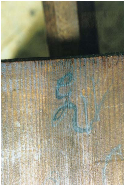
Great Stopped Diapason G# mark at top of pipe: 1768
